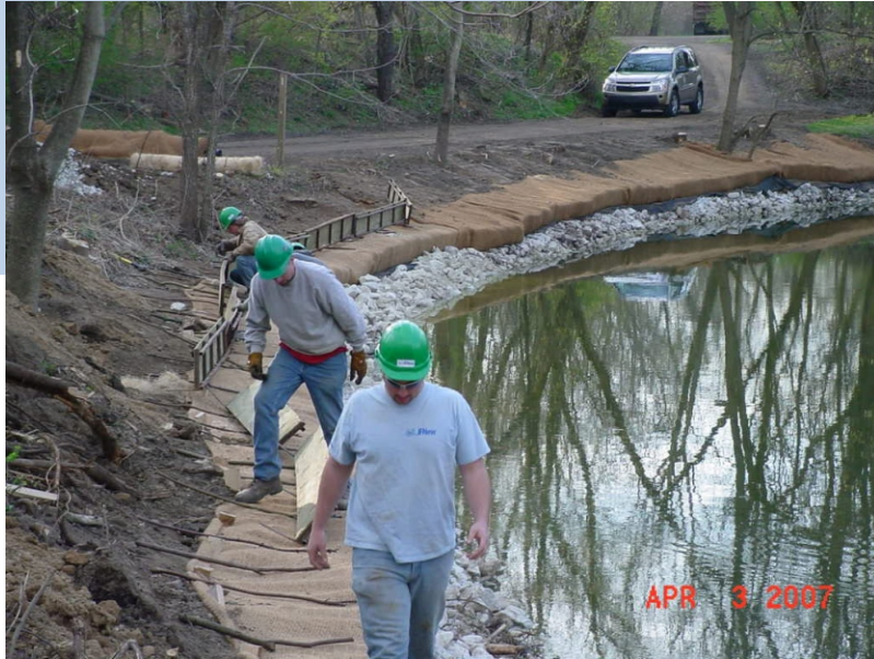
^ Installing erosion mat
